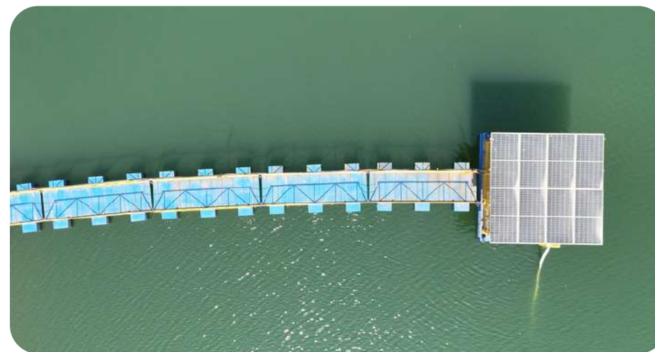
Floating Solar Pumps
