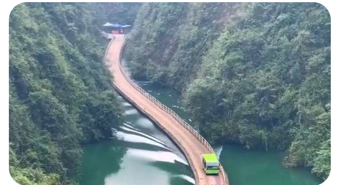
Floating walkway & Bridge
